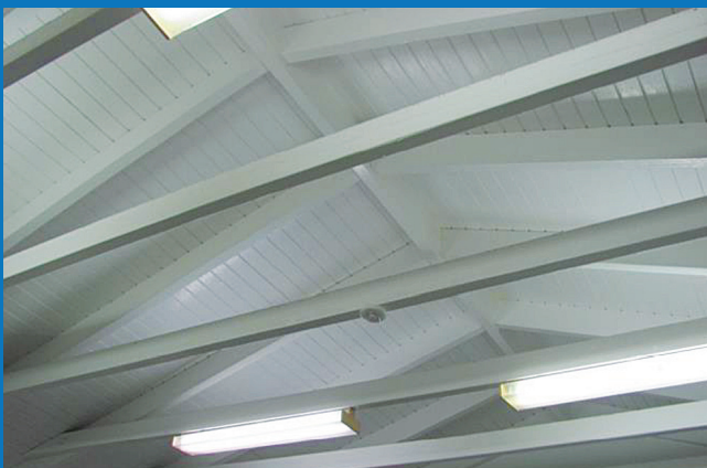
■ LIGHTING IN NEW BLOCK APPEARS ADEQUATE
