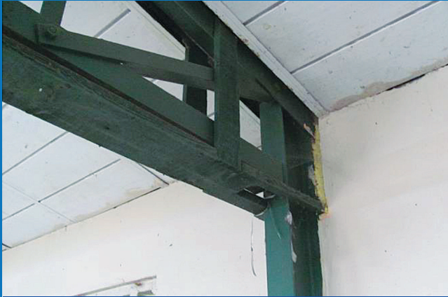
■ STEEL TRUSSES WITH TIMBER FALSE CEILING
