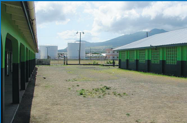
■ PETROLEUM STORAGE FACILITY ADJACENT TO SCHOOL
