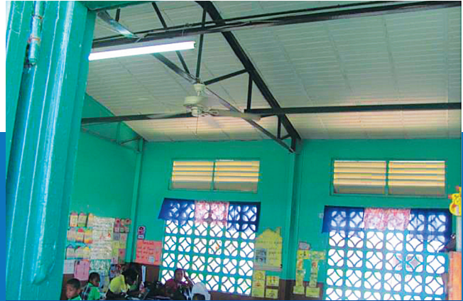
■ STEEL TRUSSES WITH TIMBER FALSE CEILING
