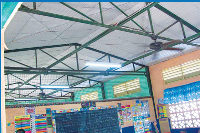
■ STEEL TRUSSES WITH TIMBER FALSE CEILING
