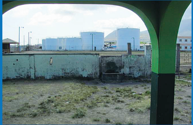
■ PETROLEUM STORAGE FACILITY ADJACENT TO SCHOOL
