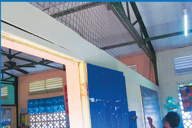
■ STEEL TRUSSES WITH TIMBER FALSE CEILING
