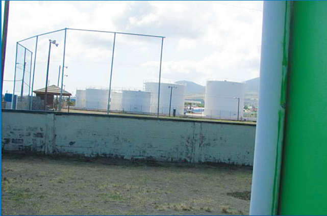
■ PETROLEUM STORAGE FACILITY ADJACENT TO SCHOOL
