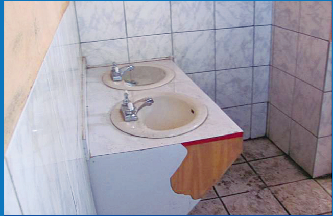
■ INTERIOR VIEW - TOILET BLOCK
