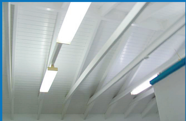
■ LIGHTING IN NEW BLOCK APPEARS ADEQUATE
