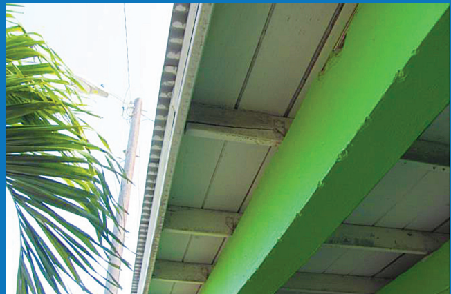
■ TOILET ROOF STRUCTURE OF TIMBER
