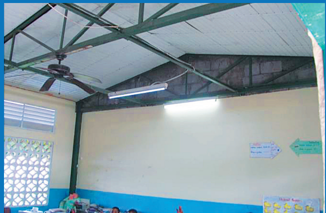
■ STEEL TRUSSES WITH TIMBER FALSE CEILING
