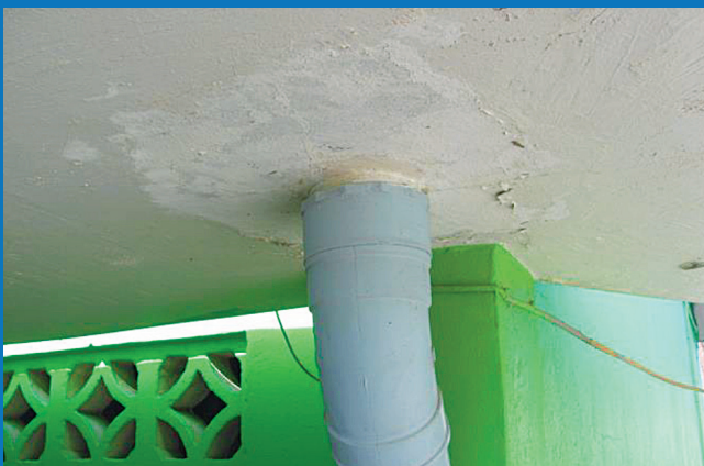
■ RECENT REPAIRS TO ROOF DRAIN
