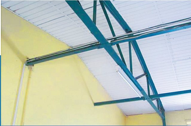
■ STEEL TRUSSES WITH TIMBER FALSE CEILING
