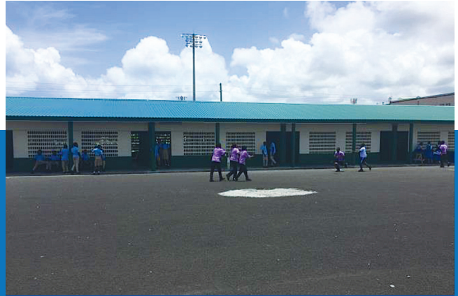
■ BUILDING WITH VENT BLOCKS - NEW ROOF
