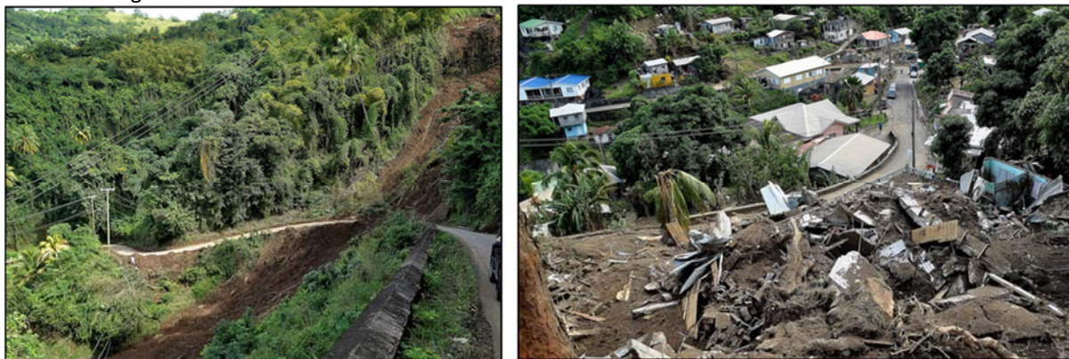
Figure 4-10: Landslides along the Leeward road, Left: landslide near Upper Vermont village, right: at Rose Bank.
