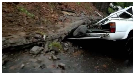
Figure 4-11: Landslide pushing a retaining wall over which killed one person in a vehicle at Hope, St Andrew, November 5, 2015
