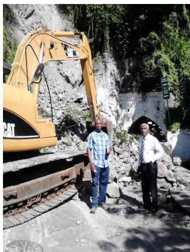
Figure 4-10: Clean-up works for the landslide/rockfall that blocked the entrance to the Sendall tunnel in September 2014
