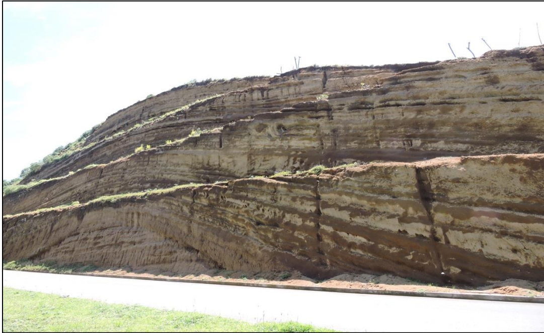
Figure 33: St Vincent, slope showing differential weathering due to lithological heterogeneity, east coast (Direction of view 035 degrees).
