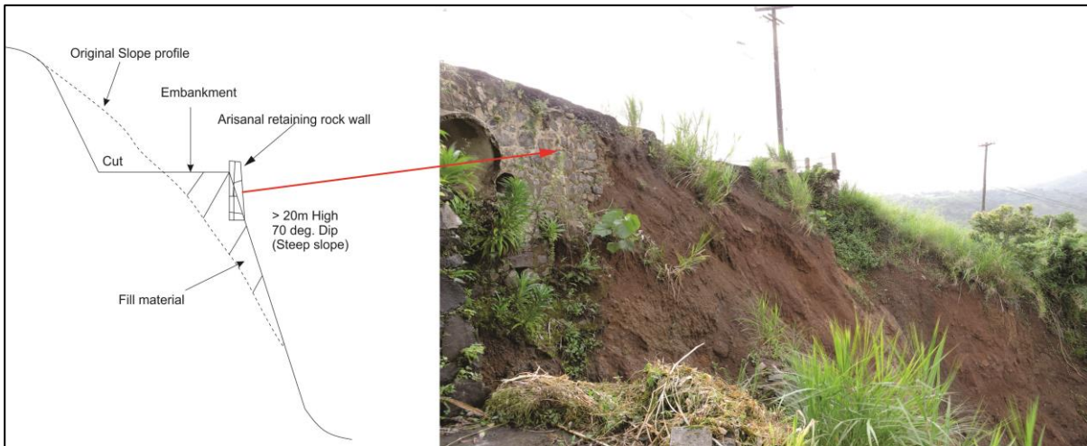
Figure 28: Belmont embankment showing the retaining rock wall (St Vincent).
