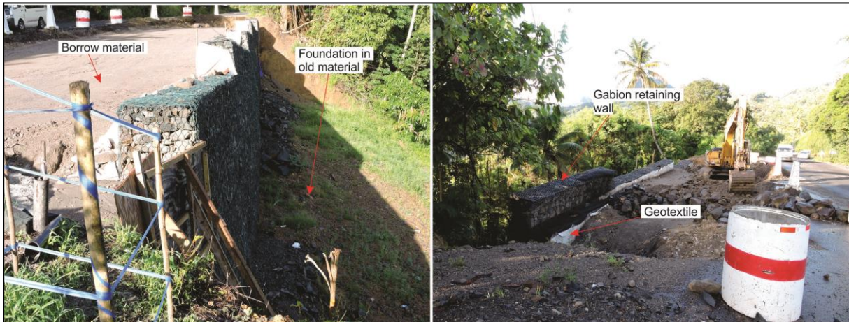
Figure 17: St Lucia, Barre de l'Isle embankment under rehabilitation (photo: Mulenga, 10/10/2014, 07:20 am).
